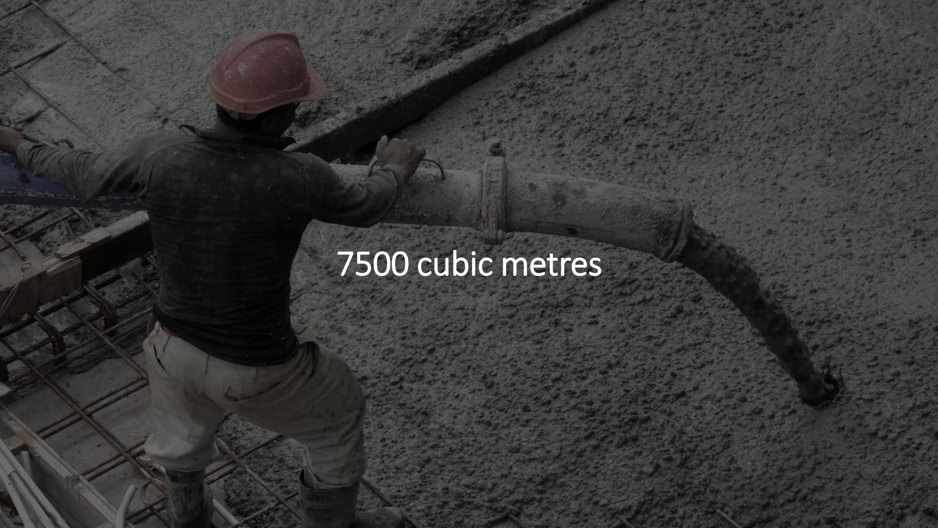
A black and white photograph showing a construction worker from behind, wearing a red hard hat and safety harness, operating a concrete pump. The worker is positioned on a metal grating over a rebar reinforcement mesh. A thick stream of concrete is being pumped from a hose attached to the pump truck into a large, flat, textured concrete surface. The background shows more of the construction site with other equipment and materials.
