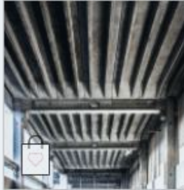
Rippenplatte Stahlbeton / L=5.79m,B=1.495m
