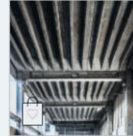
Rippenplatte Stahlbeton / L=6.84m,B=1.495m
