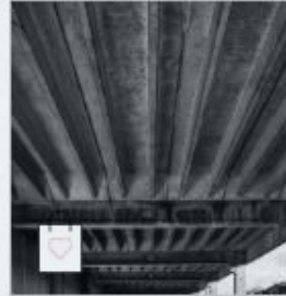
Rippenplatte Stahlbeton / L=5.99m,B=1.495m
