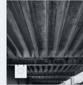
Rippenplatte Stahlbeton / L=8.97m,B=1.495m
